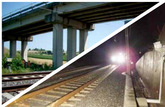
Monitoring tracks under overpasses or outside tunnels
